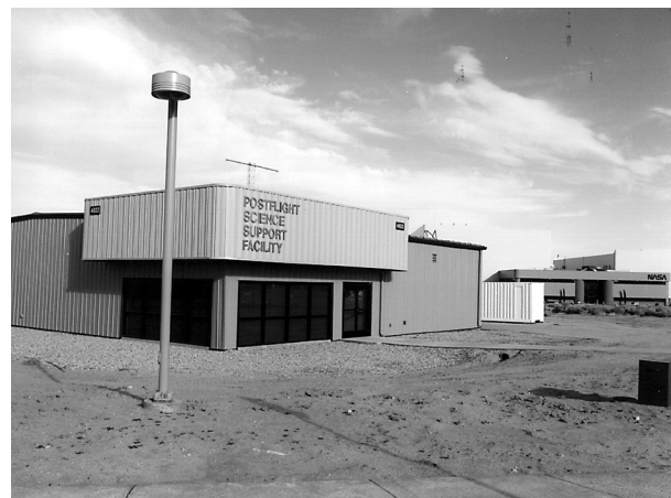
Figure 7-1. PSSF at Dryden.
